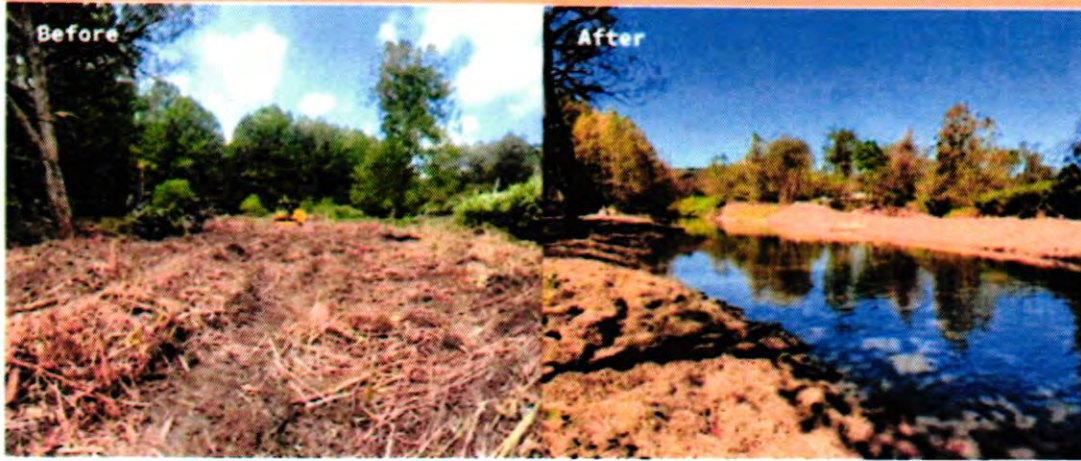
Before and After of the Oquaga Creek Restoration Project
